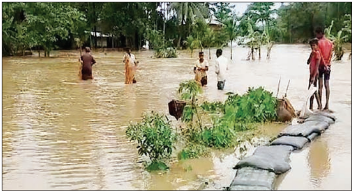
Sarma posted on X. Road connectivity of Cachar, Karimganj and Hailakandi districts of Barak Valley with other parts of the state and the northeast region has been affected with vehicles stranded, following 20 metre-stretch of the National Highway-6 being washed away by heavy rain in Lumslum area of Meghalaya. Cachar is the worst affected with 1,12,246 people reeling under the deluge, followed by 37,000 in Karimganj, 22,058 in Hojai and 14,308 in Hailakandi. A crop area of 3238.8 hectares has also been submerged, while 2,34,535 animals have been affected. The Brahmaputra and Barak rivers along with their tributaries are flooding above the danger mark at several places in the flood-hit districts. Altogether, 35,640 affected people have taken shelter in 110 relief camps (CONTD. ON PAGE-2)
