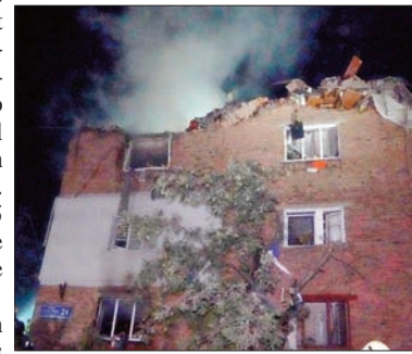
Damage from missile strikes in Kharkiv.
