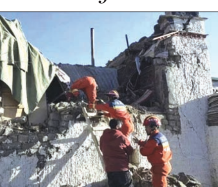
BEIJING, Jan 7: A 6.8-magnitude earthquake struck near one of Tibet's holiest cities on Tuesday, killing at least 95 people and injuring 130 others with tremors also shaking buildings and forcing people to run to the streets in neighbouring Nepal. According to regional disaster relief headquarters, the quake jolted Dingri County in Xigaze in Tibet Autonomous Region in China at 9:05 am Tuesday (Beijing Time). The US Geological Service, however, put
