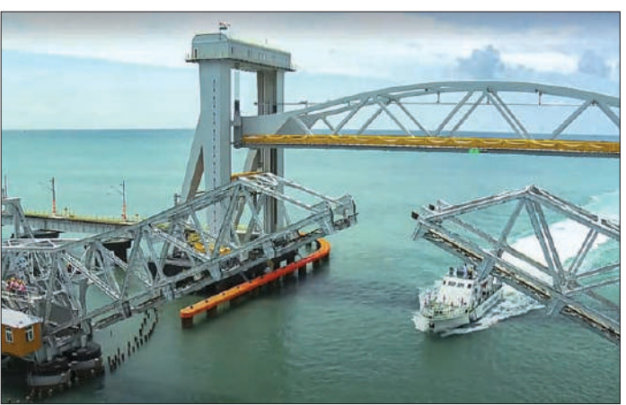
Spanning 2.08 kilometers, the bridge comprises 99 spans and a 72.5-meter-long vertical lift span that can be raised up to 17 meters, allowing the smooth passage of large ships while ensuring seamless train operations. The bridge features stainless
