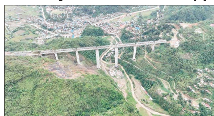
Featuring a configuration of 1x71.5m + 5x106m + 1x71.5m + 1x30m steel spans, the bridge's design is tailored to withstand the region's complex terrain and climatic challenges. It traverses hilly landscapes and deep valleys, underscoring the engineering innovation and meticulous planning behind its construction.
