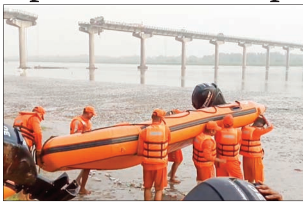
the bridge collapse.
