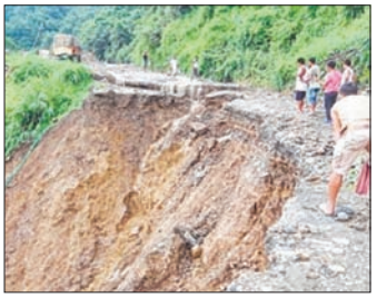
KOHIMA, Aug 25: A massive landslide on NH-2 between Nagaland capital Kohima and Wokha town completely blocked vehicular movement on the busy route on Monday.
