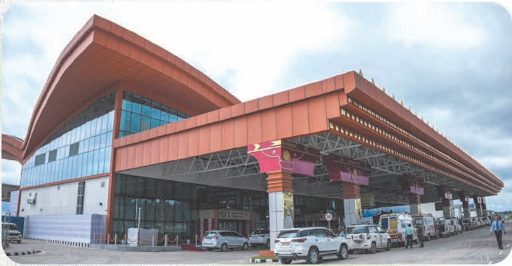
New Terminal at Donyi Polo Airport, Hollongi Delivered on 04 September 2025
