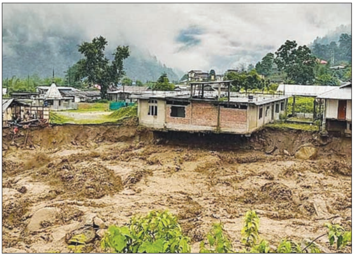
rainfall in parts of Arunachal Pradesh over the next 24 hours till Monday morning, prompting the state government to issue an alert and urge people to remain vigilant. The body of Saurabh Kumar Kharwar was found near Hawa Camp, which is around 35 km from flood-hit Poosa in Keyi Panyor district, State Disaster Management Secretary Dani Sulu said, adding a rescue team has been dispatched to retrieve the mortal remains. Five people went missing after a flash flood, triggered by incessant rainfall, struck Keyi Panyor district on Wednesday morning. With the latest recovery, three people have been confirmed dead, while two others remain missing. The body of a 35-year-old woman was recovered on Wednesday, while another woman's body was found on Saturday. Search operations entered the fifth day on Sunday, with a rescue team using rafts from the dam side of the Panyor Lower Hydroelectric Project and another ground team searching for the two missing persons who were swept away from the NEEPCO Colony, another official said. Relief and rescue efforts have also been intensified in the affected region. An additional 23 personnel from (CONTD. ON PAGE 2)
