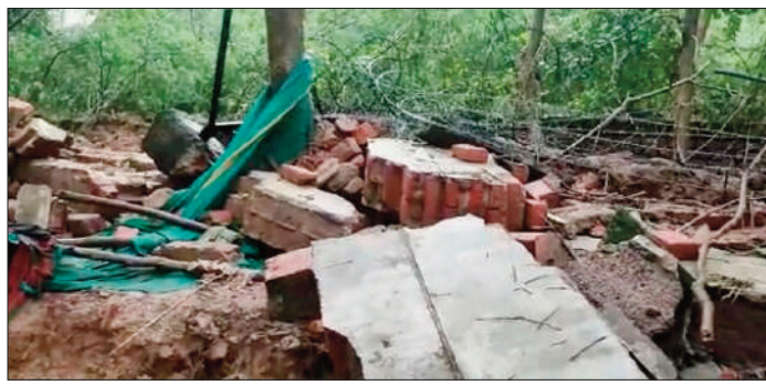
PRATAPGARH/BARABANKI/SAHARANPUR (UP), Aug 6: Six members of a family, including two infants, were killed after a nearly century-old house collapsed during heavy rains in Uttar Pradesh's Pratapgarh district early Thursday, police said.
